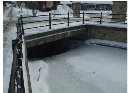
The control structure at Drummond Street
