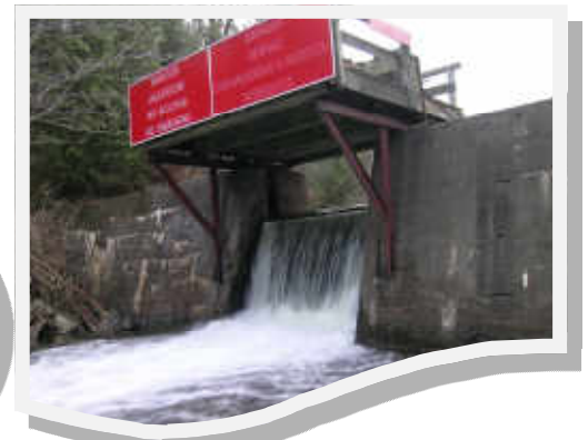
We monitored the Update of the Bolingbroke Dam
