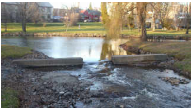
Participating in modifications to Haggart Island Dams and monitoring progress.
