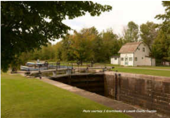
Upper Beveridge Lock
