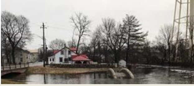
View from Bath House at swimming area looking east on stone bridge
