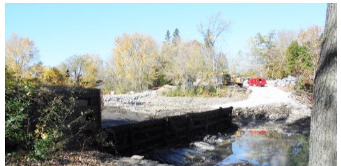
The dry Haggart Dam
