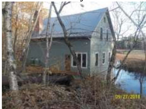
Rear View of Fream Mill
