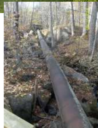
Pipe dam to Mill
