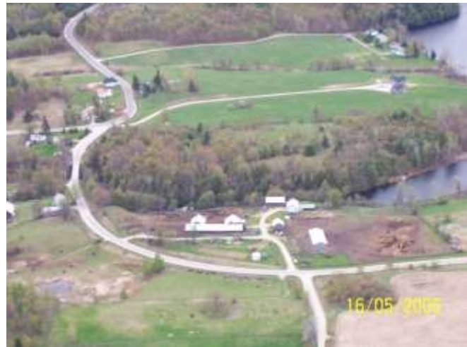
Bolingbroke Dam site today (Bobs Lake at right)
