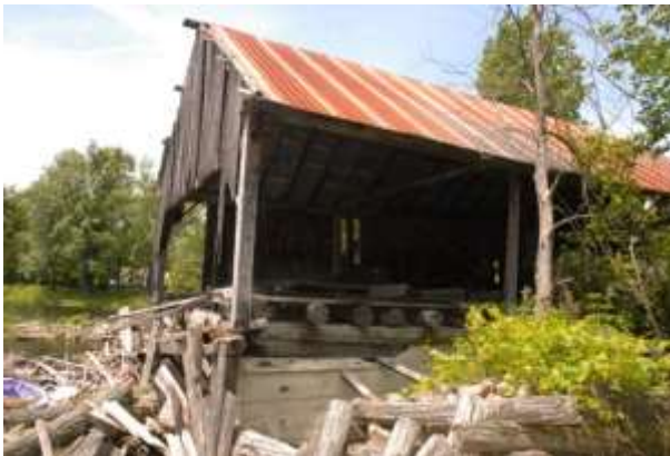
Log Chute into Ritchie Mill (David Zimmerly)
