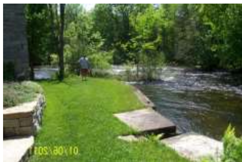
McCabe Grist Mill Shore Foundation & Sluice Area
