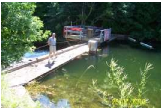
Bolingbroke Dam, before its removal, and construction of new dam upstream, in 2018/2019
