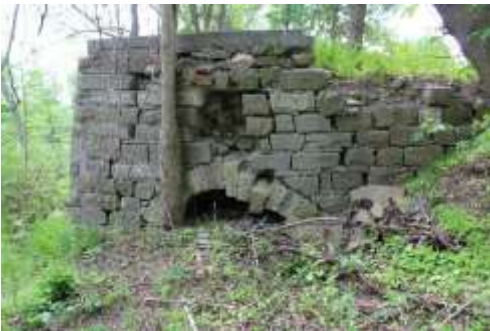
Ruins of the Grist Mill, beside the main dam (2016)
