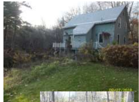
Front View of Mill
