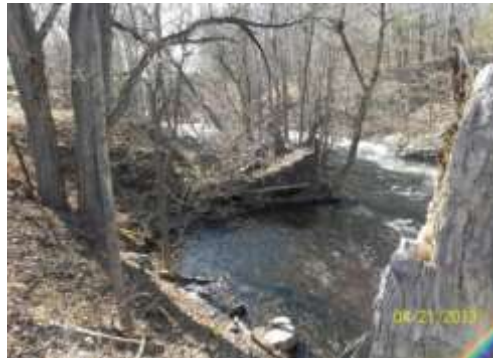
Foundation of the cloth and carding mill, behind the Maberly Fall River restaurant.
