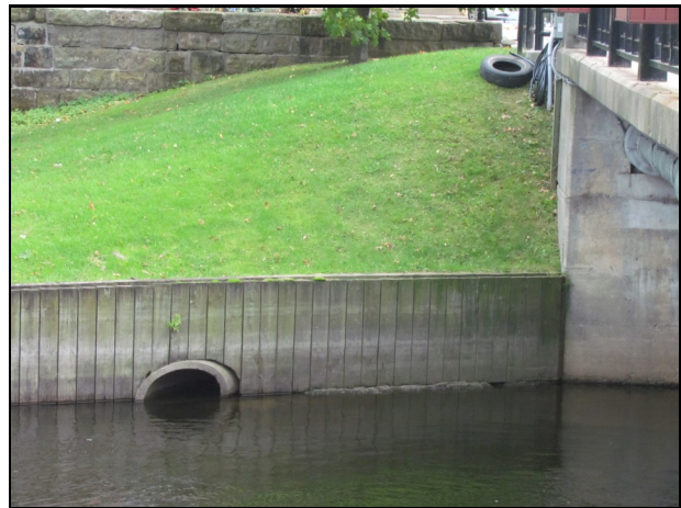
Site 2 — Gore Street Bridge
