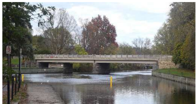
Drummond Street Bridge, Post-1981 (Hamilton Spectator)
