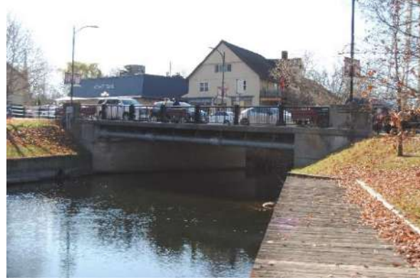
Big Tay Gore Street Bridge, 2022 (Ron W. Shaw)
