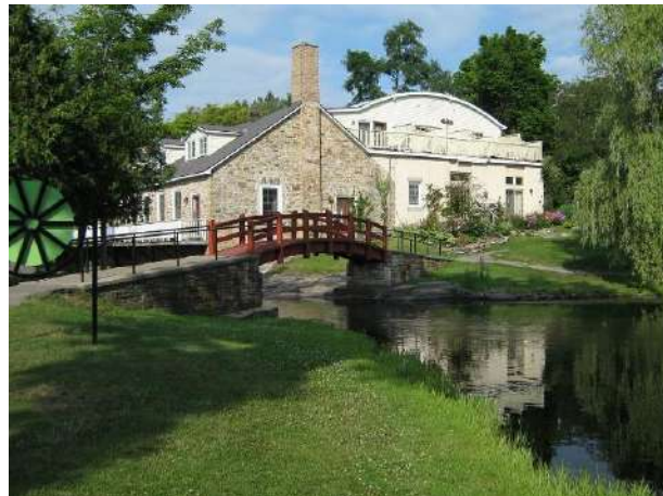
Douglas Cavers Bridge, 2022 (Ron W. Shaw)
