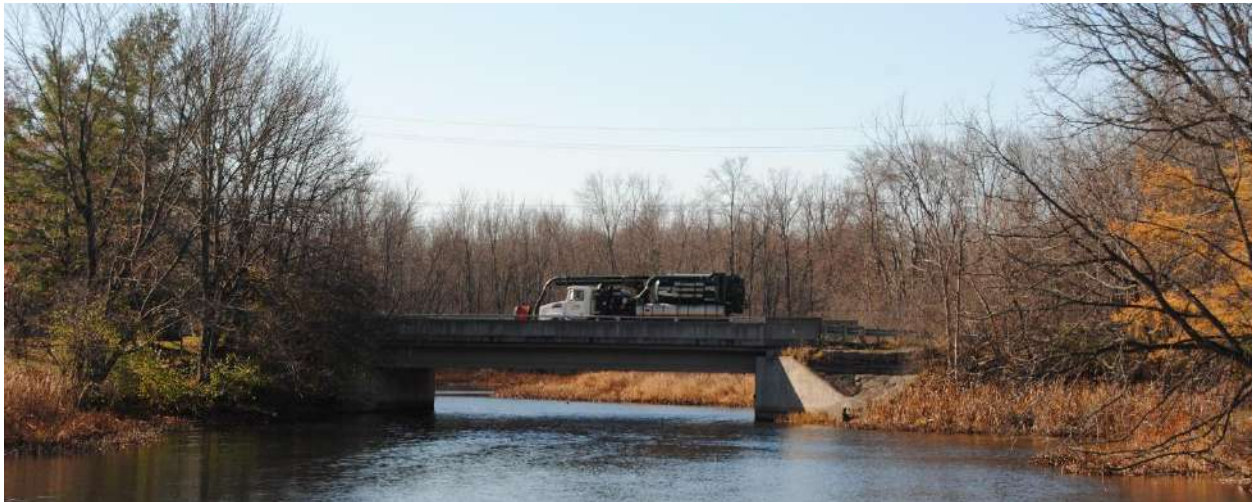
Rogers Road Bridge, 2022 (Ron W. Shaw)
