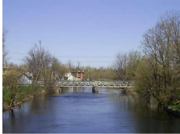
Beckwith Street Bridge, 2011 (Ken Chaplain)
