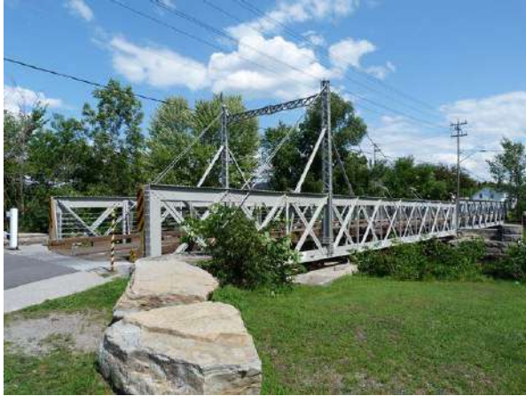
Beckwith Street Bridge, 2013 (Holth & McOmber)
