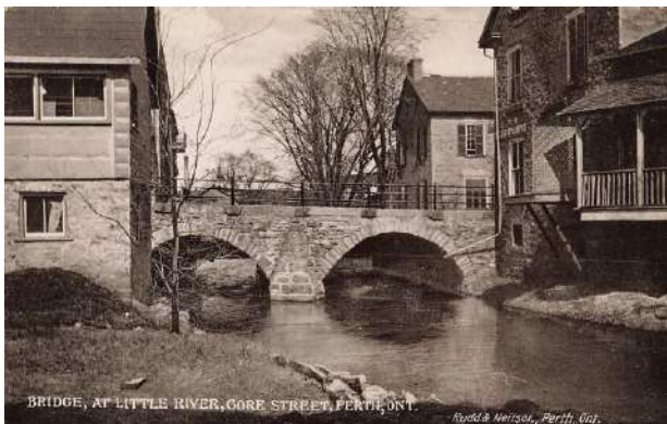
Little Tay Gore Street Bridge, c1910 (Rudd & Neilson)
