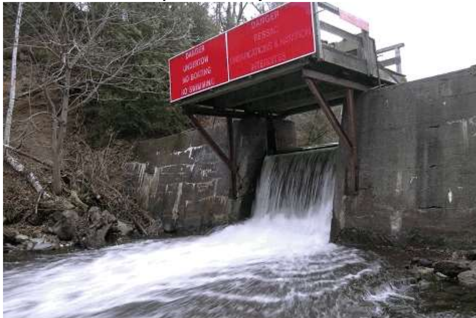
Bobs Lake Dam
