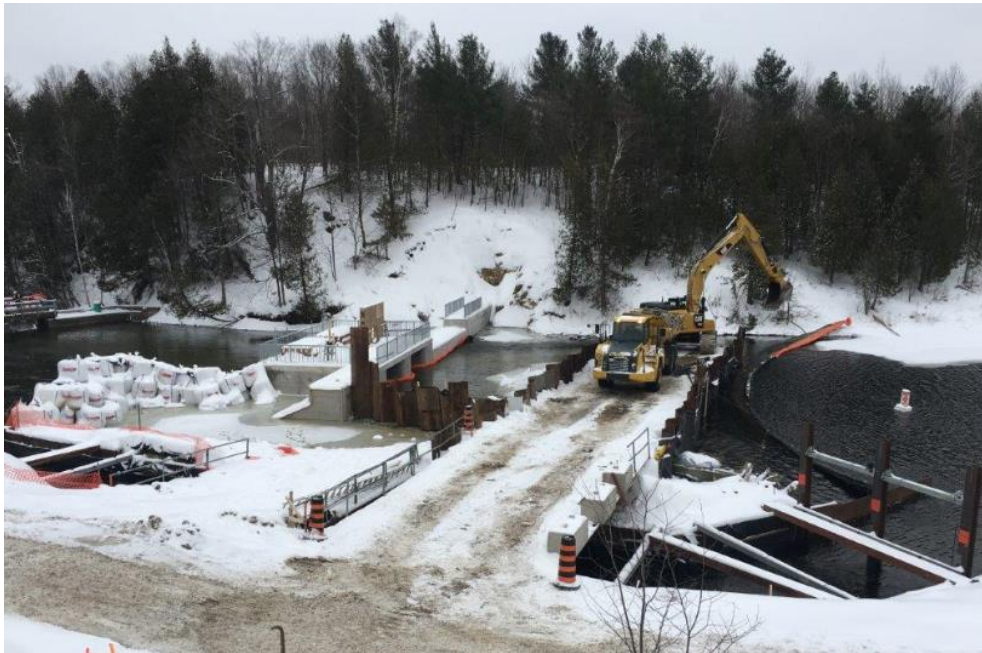
Removal of a cofferdam at Bobs Lake Dam
