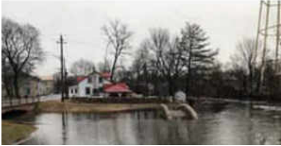
Mill St. swimming area in flood
